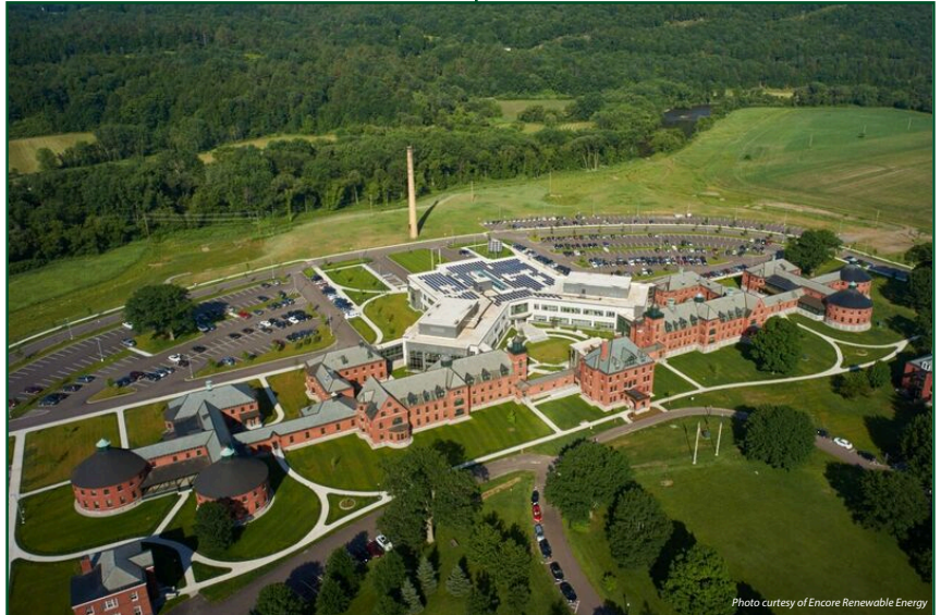
Photo courtesy of Encore Renewable Energy
