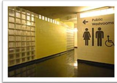
Careful design of wall locations will allow restroom entrances without physical doors Courtesy of: The Full Wiki
