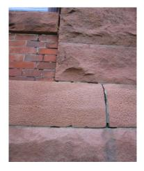
original red ochre tinted lime putty cement was disregarded. It also appears that the building windows have never been properly restored; the storm windows that were added are in serious need of repair causing further infiltration issues. In the 1970's the original slate roof was removed and replaced with asphalt shingles, which are currently failing.
