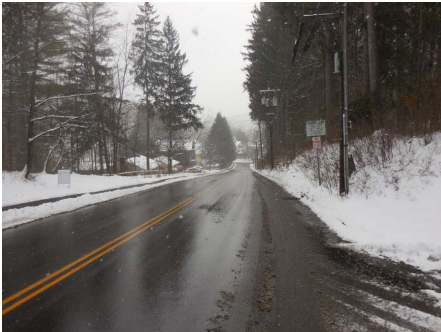
Terrace Street - Looking Southeast
