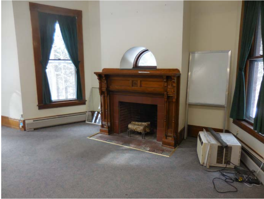
First Floor Office Area
