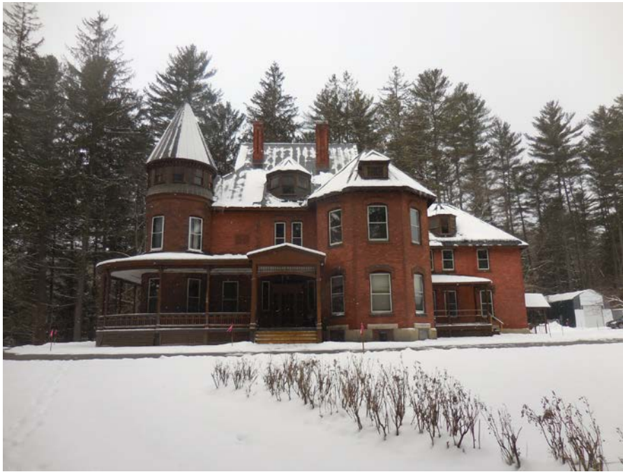
Subject Building - Looking Westerly
