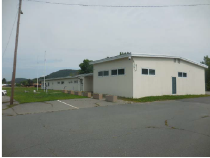
Front of Building
