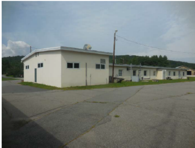
Back of Building
