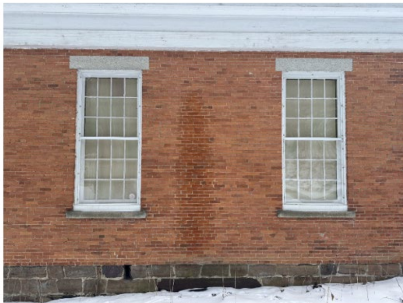
Examples of windows (all 8 windows will be receiving new storms)
