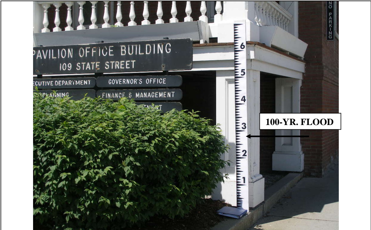
Montpelier Complex – 109 State Street (Date: June 2006)
