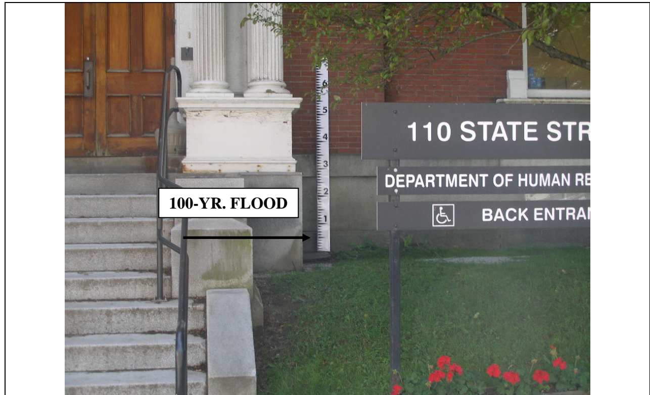
Montpelier Complex – 110 State Street (Date: June 2006)
