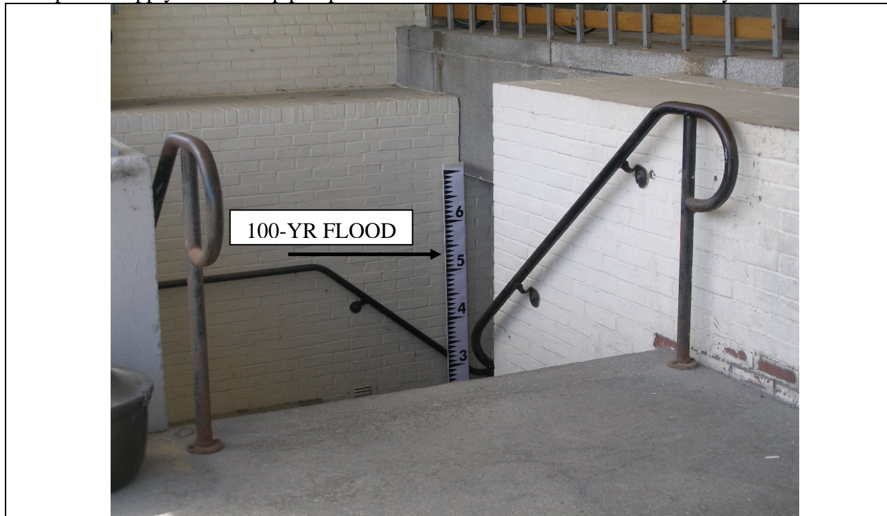
Montpelier Complex – 120 State Street Date: June 2006
